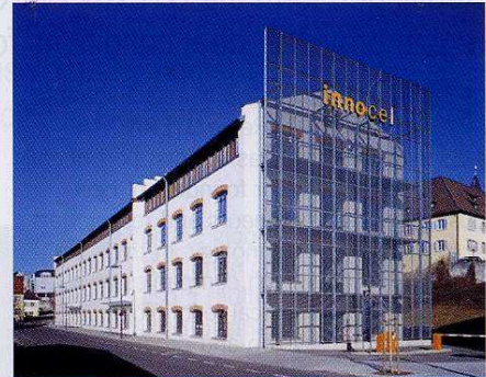
Innocel is based in a renovated historical building, now housing 30 companies
